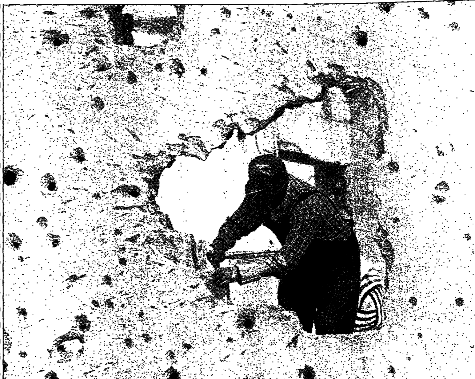
A man repairs his house in a once front-line suburb. Now the windows will be smaller and will not face the mountains. PHOTOGRAPH: DANIL KRISTANOVIC
